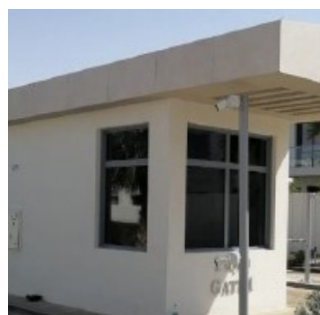
Modification of Gatehouse glass pane to tinted sliding windows
