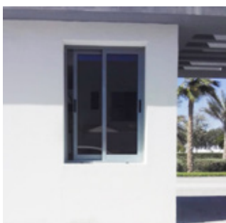
Modification of Gatehouse glass pane to tinted sliding windows
